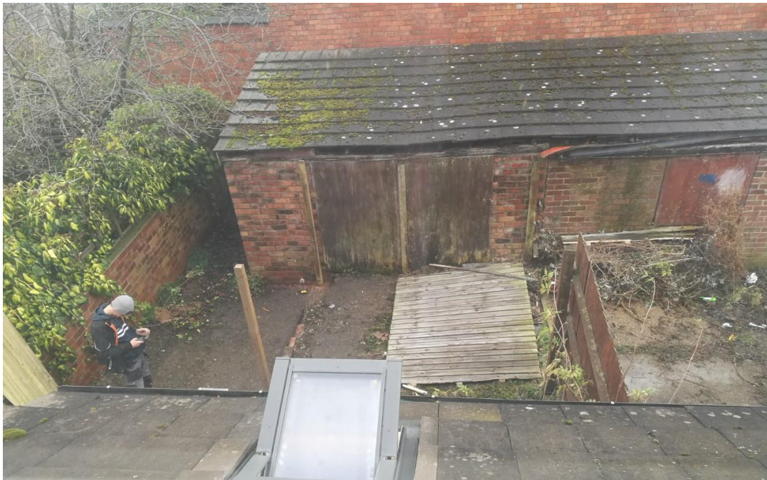
Applicant Photo taken looking down into yard before works commenced to rear yard
