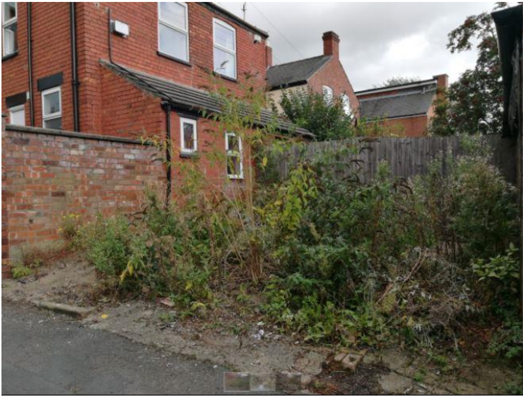
Applicant Photo taken before works commenced to rear yard.
